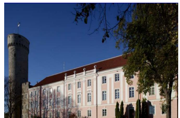
Heritage buildings present particular challenges that require a balance between preservation and sustainability. The Parliament of Estonia
